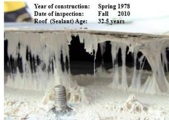
Any sealant used in latent metal construction details should be intended for long life as it is not easily repaired or replaced without potential damage to panels or other parts. Such details should accommodate expected movement through the design of the joint itself, not purely by sealant deformation.
