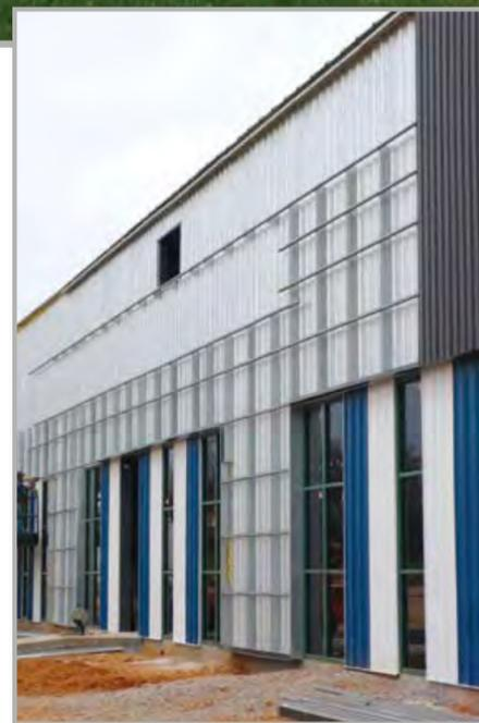
insulates buildings' inner walls by shielding them from direct sunlight during the summer. Furthermore, InSpire destratifies hot air treated at the ceilings, resulting in lower temperatures for air exhausted through the roof. InSpire consists of ATAS metal wall panels, fans, dampers, ducts and other ventilation components in conjunction with an electronic control system.
