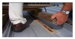
Figure 3. Roof corrosion from treated wood
