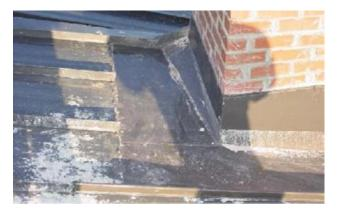
Figure 4. Cement, mortar, and related products can damage metal roofs
